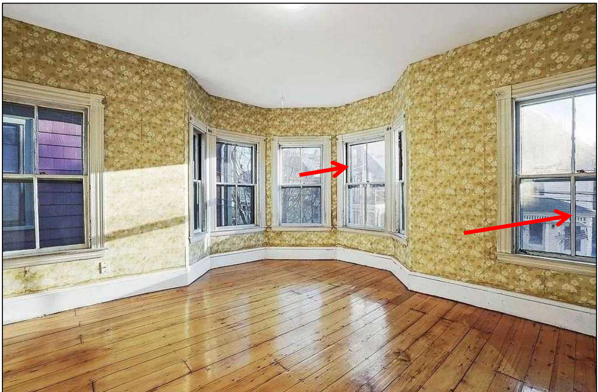
Above: Note original tracks and original wood sash and muntins.
